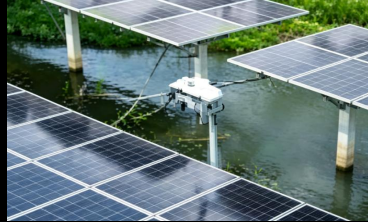
Stable Operation at Height
